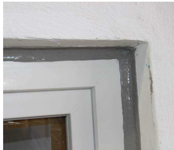
Photo 4 Top corner details of external joint
