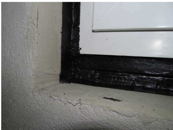
Photo 5 Bottom corner details of internal joint
