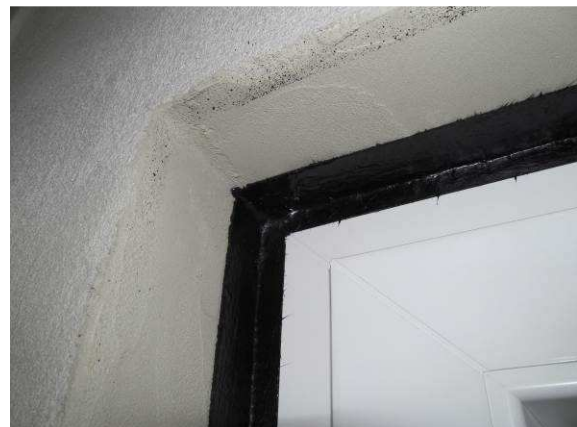
Photo 6 Top corner details of internal joint
