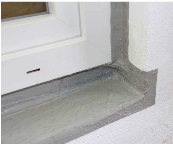
Photo 3 Bottom corner details of external joint
